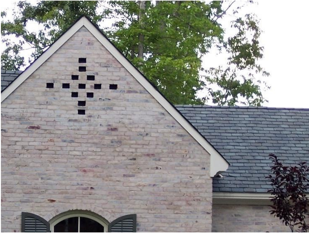
ELEVATION - Flush Rake with Decorative cornice end board as a molding stop
